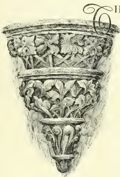
Corbel in Lower Church
